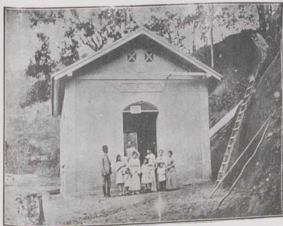
Uzina hydro-electrica — Muquy do Sul
